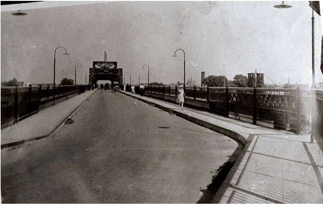
I St. Bridge ca. 1912 Looking East towards Sacramento (Photo taken from “dogleg” section.)
